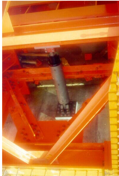
Fig. 9: Installed MHD in Seyhan Bridge
